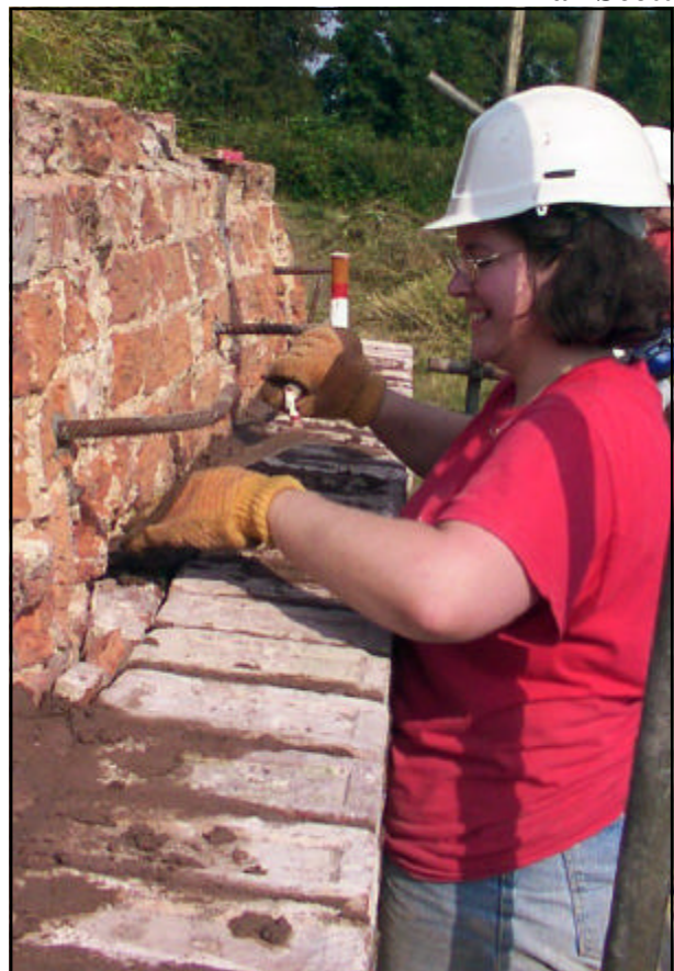
Harri T building the lower wing wall (Ed Walker)
