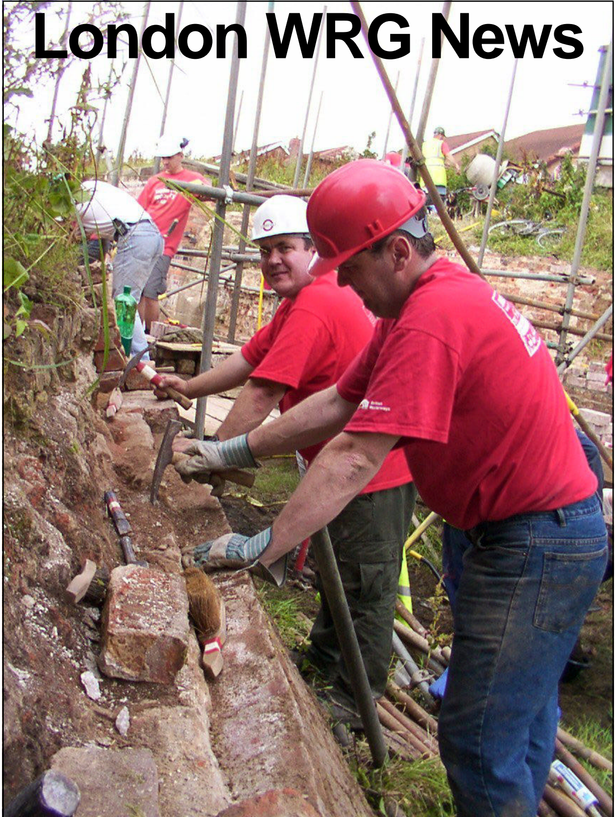
Bob and Taz cleaning up the brickwork (Derby Canal, Ed Walker)
