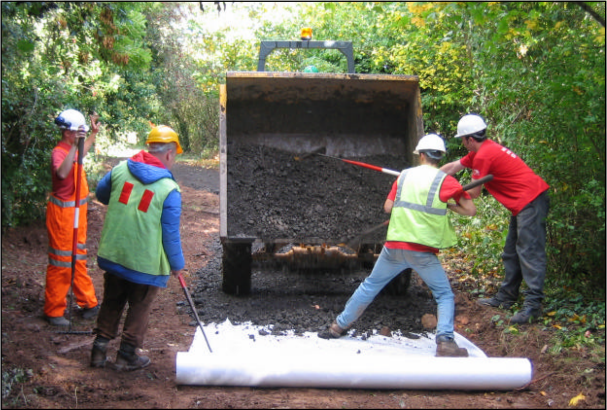
Cycleway laying on the H&G (Martin Ludgate)
