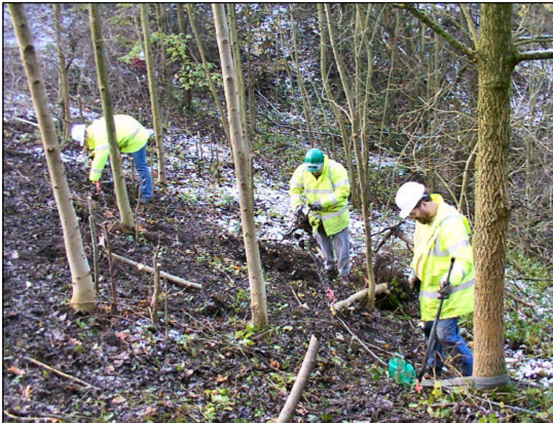
Stump pulling on the embankment (Ed Walker)
